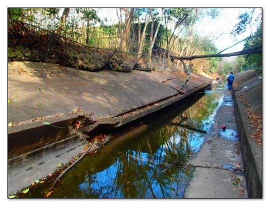
Figure 2-5: View of Concrete Pavement Damages Along Project Reach
